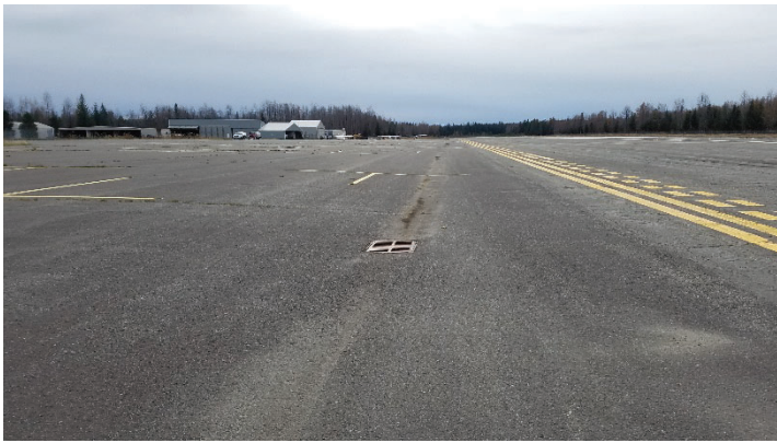
Exhibit 1-1: Gustavus Airport AFFF training area.
