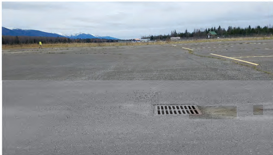
Exhibit 2-3: New fire-training location.
